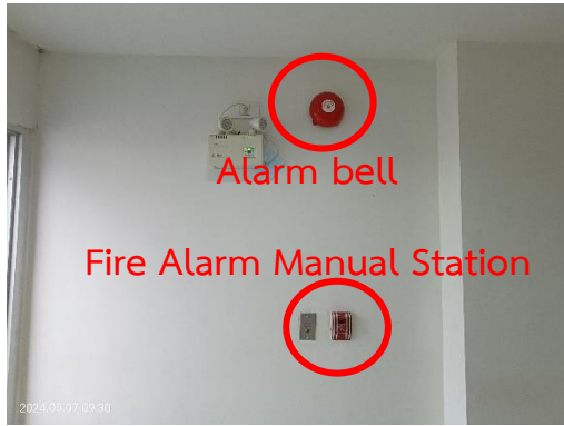
Alarm bell & Fire Alarm Manual Station
